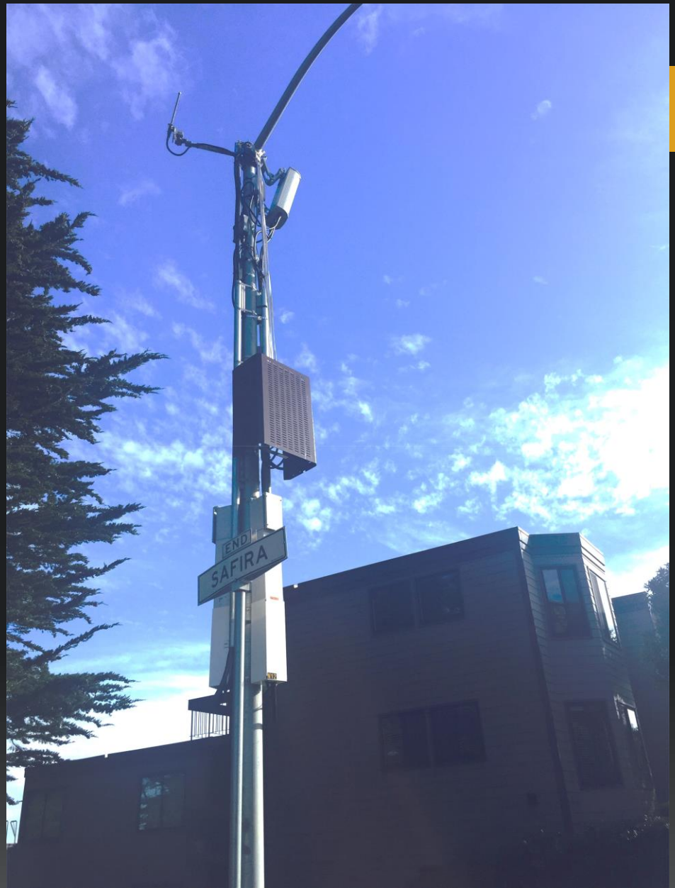
Actual Crown Castle Site. Modifications made w/o permits (whip antenna for Sprint, panel for Verizon)
