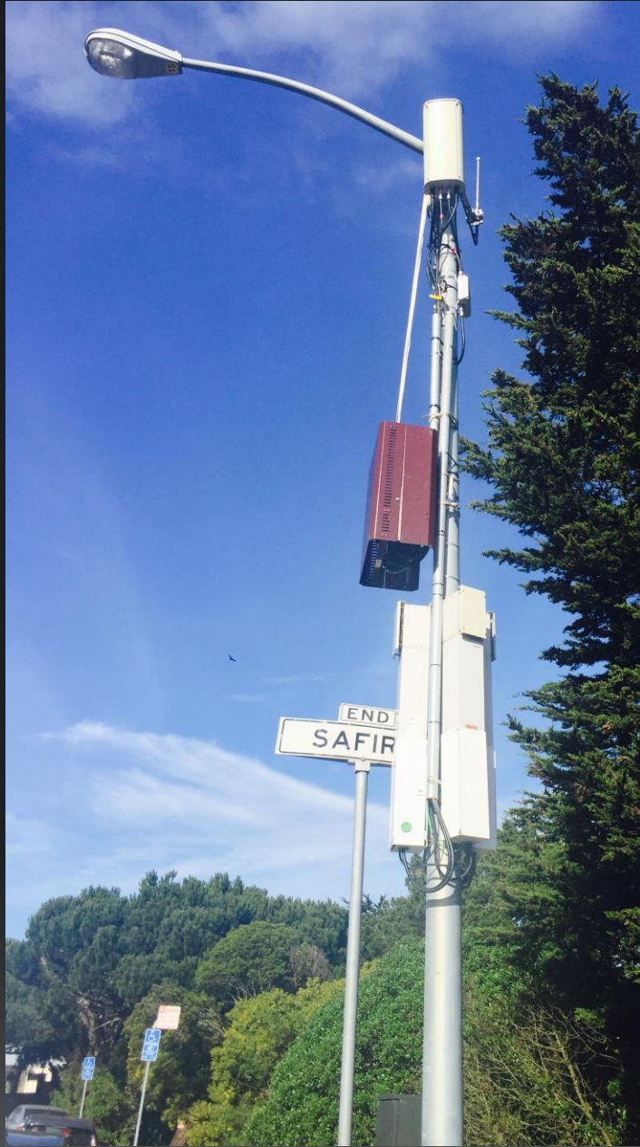
Actual Crown Castle Site. Modifications made w/o permits (whip antenna for Sprint, panel for Verizon)
