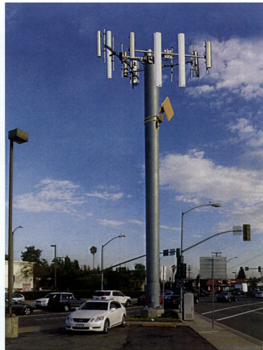
Permitted modification under AB 162 (larger pole, additional antennas, and failure to blend with surroundings)
